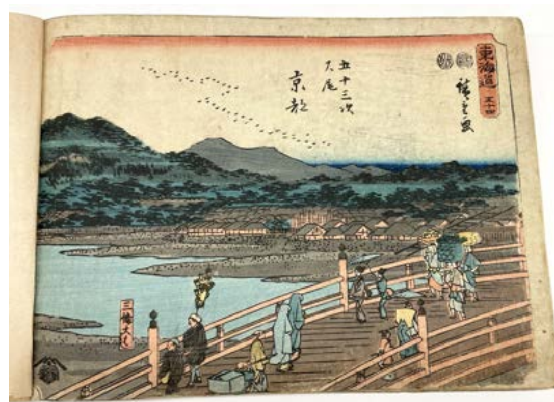
The bridge Sanjō Ōhashi in Kyoto.
